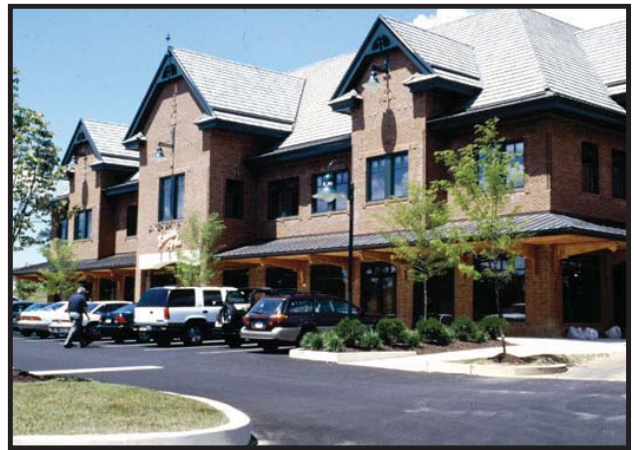
Ground Floor Restaurant and Second Floor Offices & Retail, Eagleview Town Center, PA
