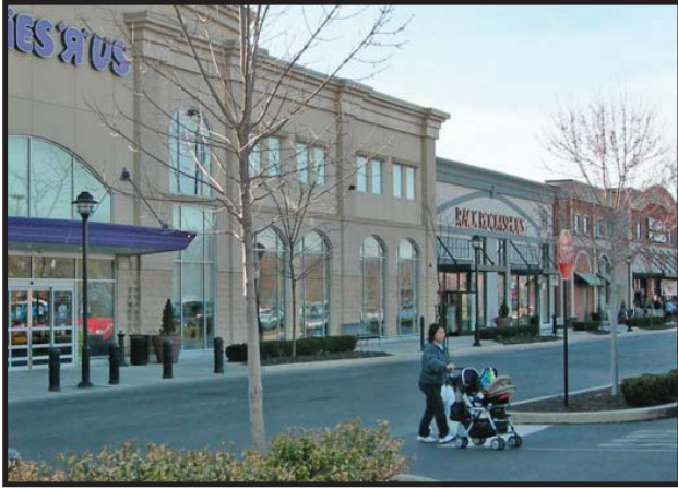
Commercial Buildings Detailed with Vertical Bays and Pilasters extending as a full vertical section, Main Street at Exton, Exton, PA
