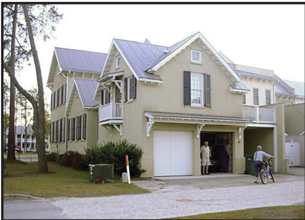
Detached Garage off Alley, Habersham, Beaufort, SC
