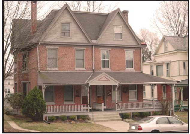
Twin Design with Gables and Front Porch, West Chester, PA
