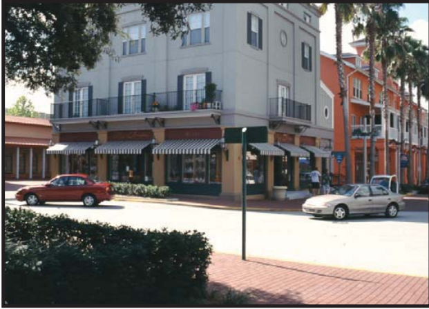
Offices Over First Floor Retail, Celebration, FL
