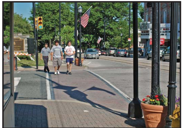
Crosswalk at Grade, Media, PA
