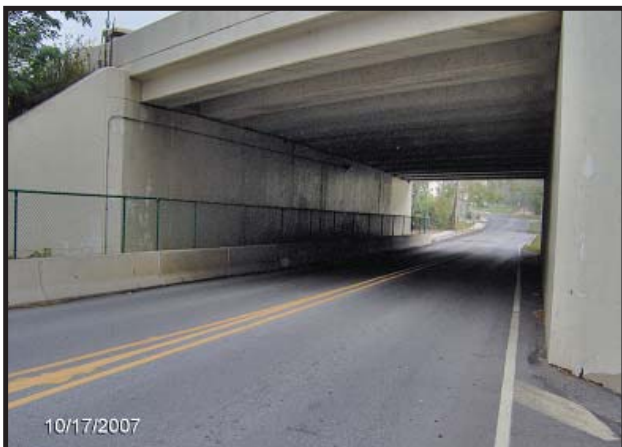
Example of Pedestrian Pathway Bell Tavern Road, East Caln Township
