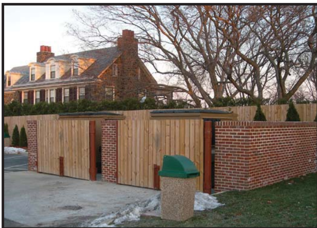
Brick Wall Enclosure of Dumpster, Claymont, DE
