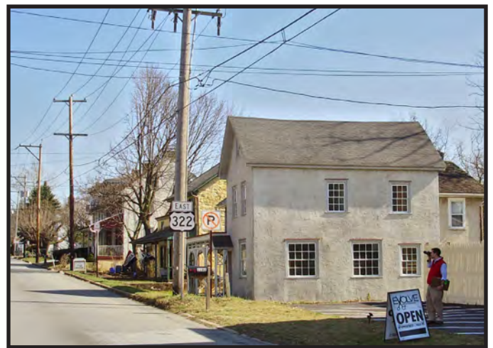
Existing buildings in alignment along Route 322.
