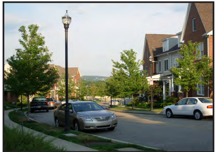
Decorative lighting and street trees installed in a grass strip along the cartway.
