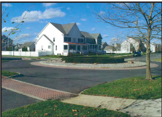
A decorative crosswalk contrasts with the cartway surface in order to promote visibility, and promote pedestrian circulation.
