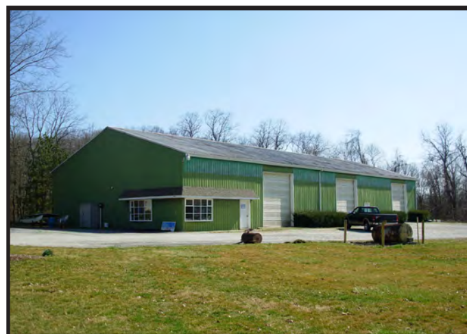
A non-historic building in Guthriesville Village that presents an opportunity for adaptive re-use.
