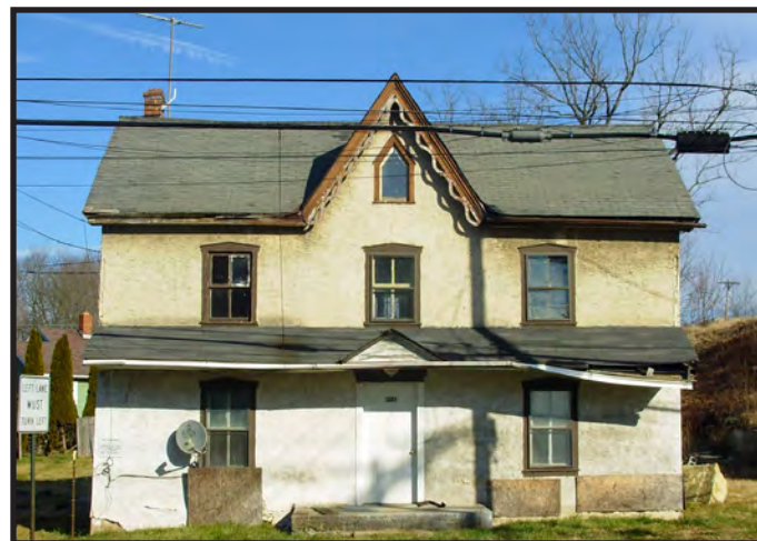
An opportunity for rehabilitation and adaptive re-use.
