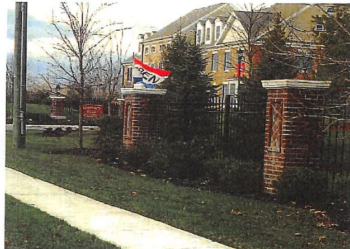
Well Maintained Streetscape Edge
