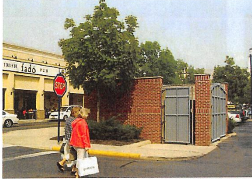
Attractively enclosed dumpster area.
