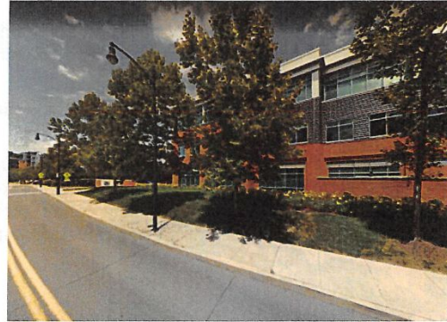
Buildings located in close proximity to the Sidewalk system.
