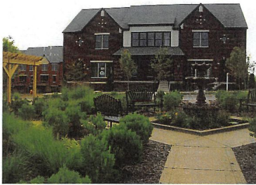
Attractively designed and maintained Public Open Space area as a link between buildings.
