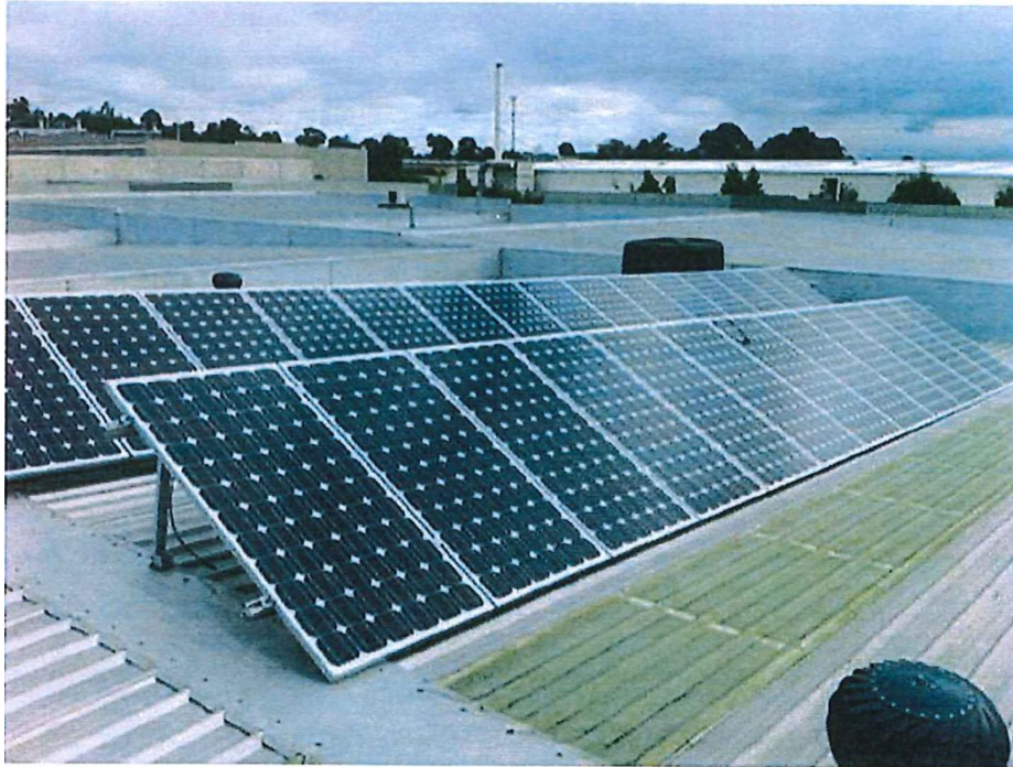
Flat-Roof-Mounted Solar Energy System (Illustration No. 3)
