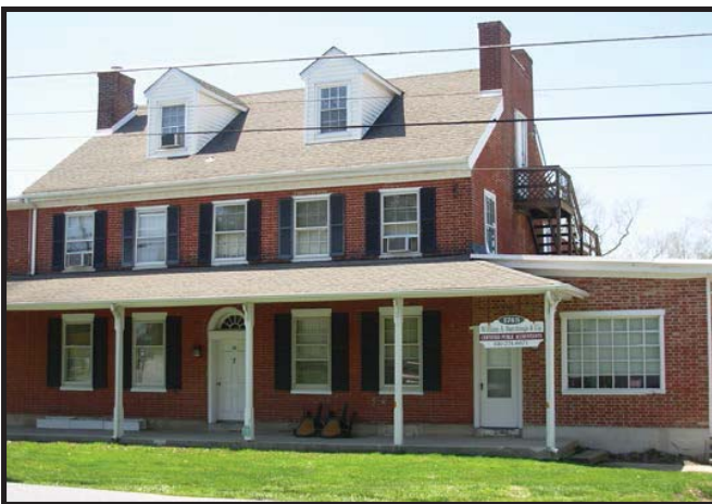
Attached Dwellings in Kemblesville
