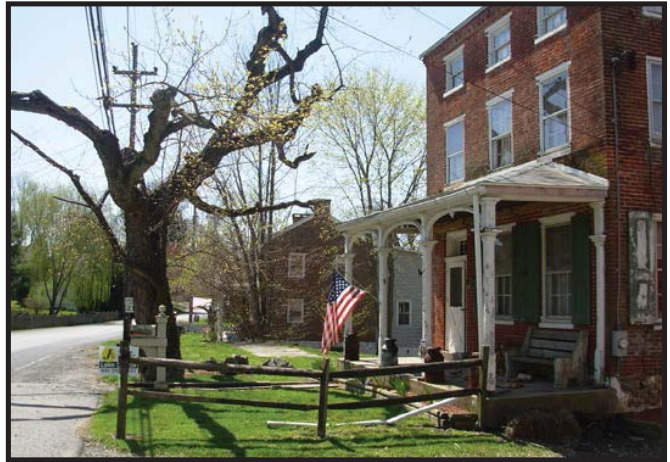
Building with Front Porch Near Appleton Road
