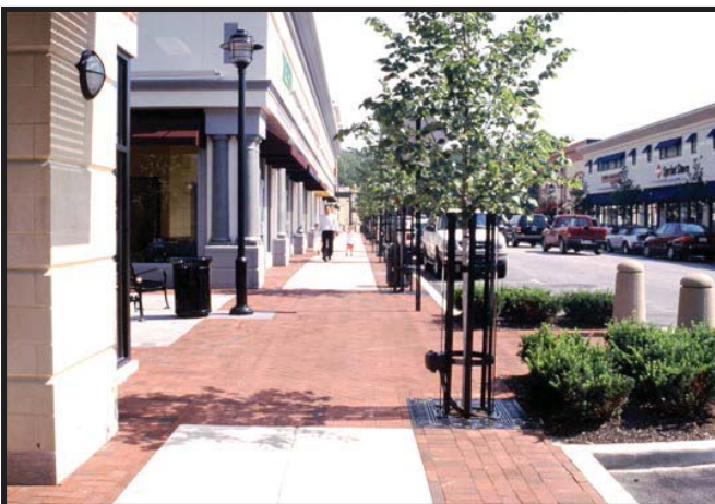
Sidewalk with Brick "Apron" at Main Street at Exton, Exton, PA
