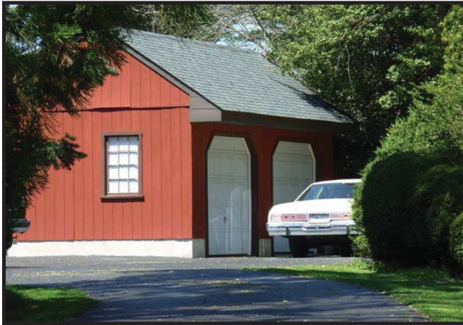
Detached Garage in Kemblesville
