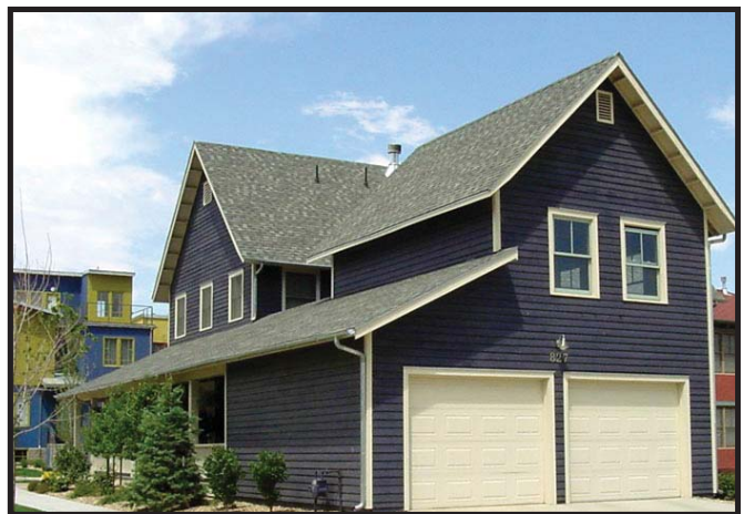
Apartment Above Garage: Longmont, CO
