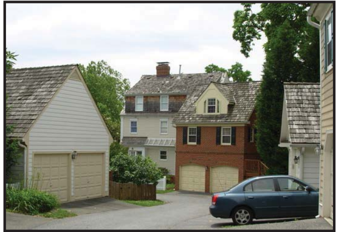
Apartment Above Garage: Kentlands, MD
