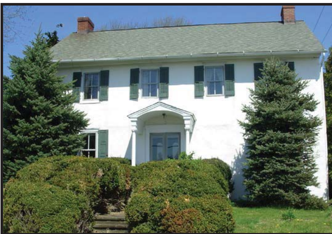
Portico in Kemblesville Village
