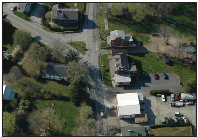
Buildings Located Close to Road, with Shallow Front Yards
