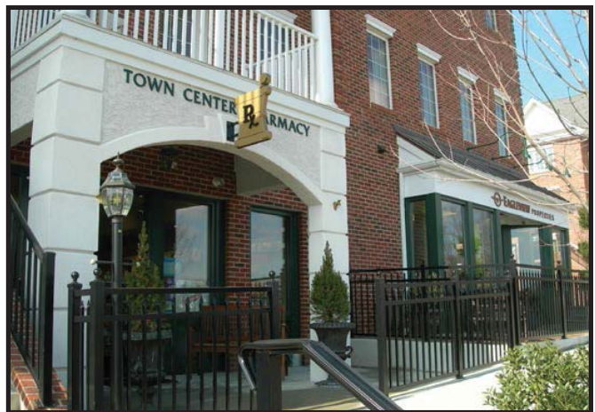
Example of Live-Work Unit, Eagleview, Lionville, PA
