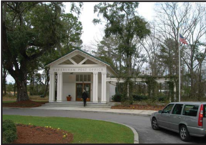
Example of a private mail facility, Habersham, SC
