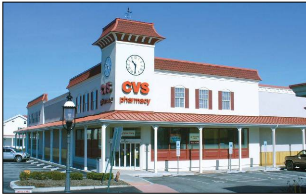
National Chain Store, Eagle, PA: Made to look distinctive, the mass of a medium sized retail store has been broken up, creating the illusion of several smaller buildings attached by a covered porch. Note the use of windows, shutters, and "clock tower" feature, extending the second floor.
