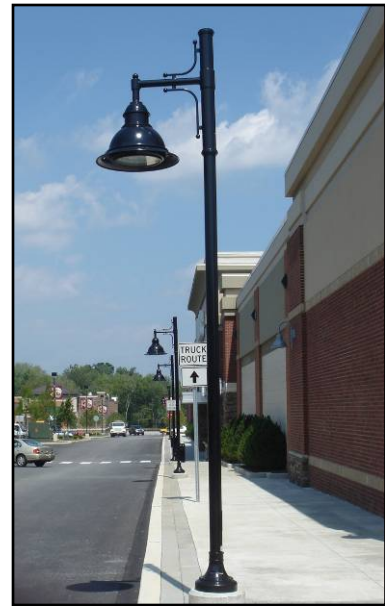
Concordville, Delaware County: Use of the DMS50 fixture on a higher pole to illuminate secondary/access roads. The same fixture and pole could be used to illuminate commercial parking areas in North Coventry Township. Further, note the use of decorative flags on the pole to enhance sense of community identity.
