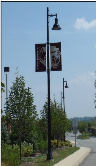
Concordville, Delaware County: Use of the DMS50 fixture on a higher pole to illuminate secondary/access roads. The same fixture and pole could be used to illuminate commercial parking areas in North Coventry Township. Further, note the use of decorative flags on the pole to enhance sense of community identity.
