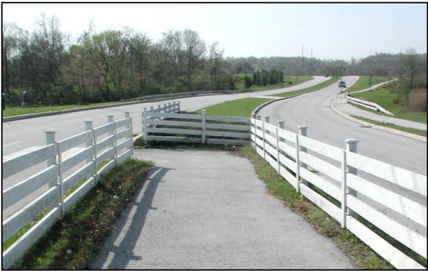
West Whiteland Township, Chester County: Close-up of the pedestrian crossing shows how this fenced median creates a safe environment for pedestrians crossing the divided road.
