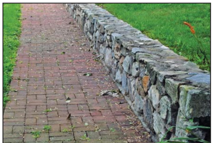
Stone Wall along Sidewalk
