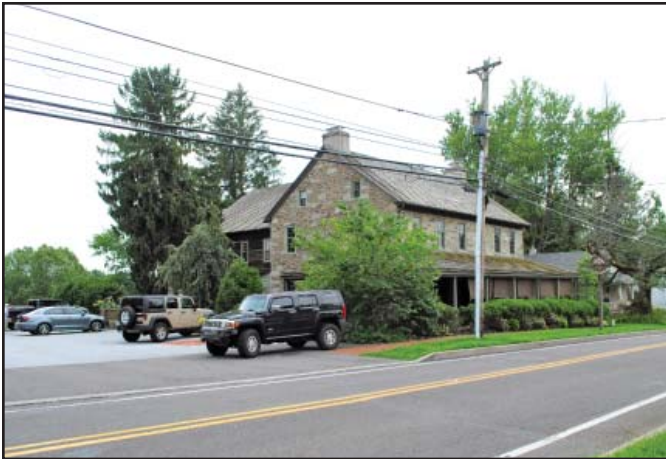
Existing Utility Poles with overhead electrical wires
