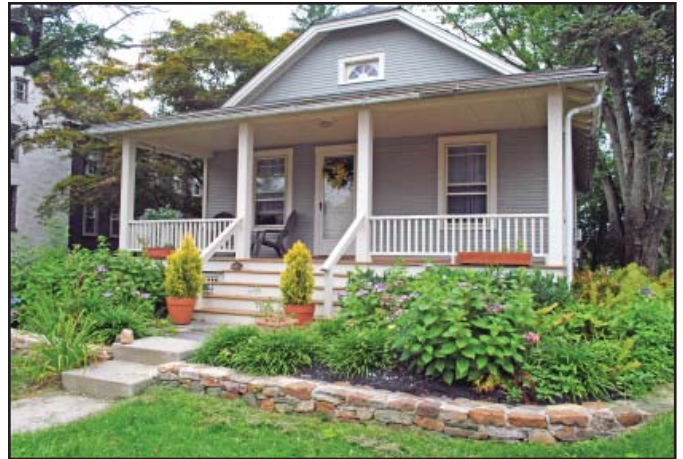
Landscaping complementing Building and Streetscape
