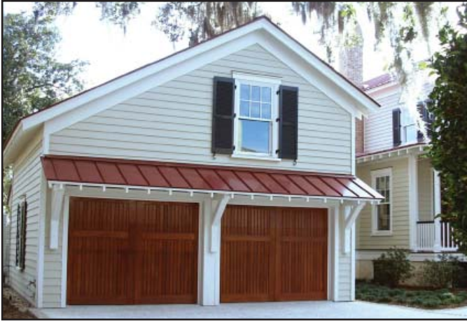
Detached Garage with complementary building materials
