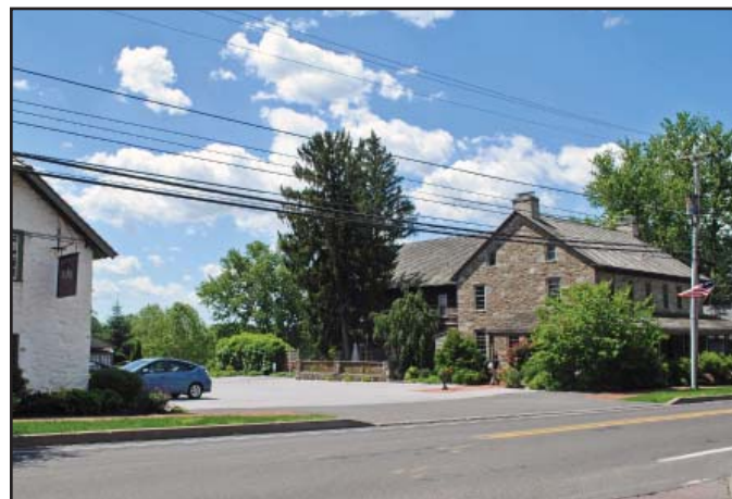
Wide Curb Cut for Restaurant
