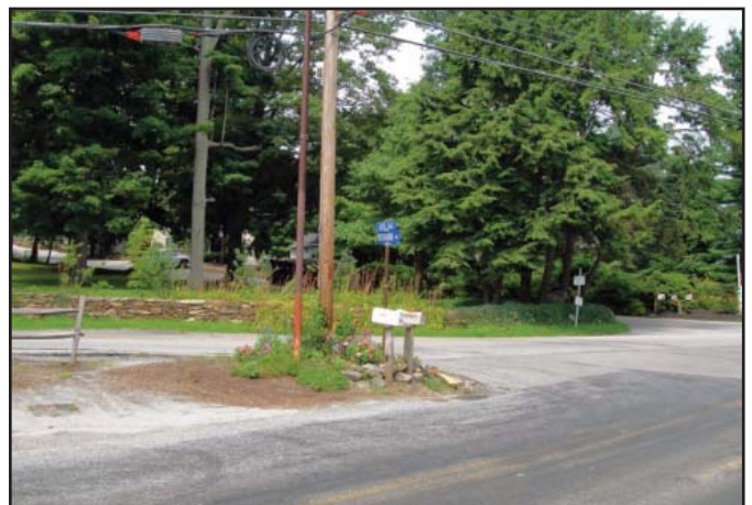
Existing Utility Pole and Wires at Strasburg and Northbrook Roads
