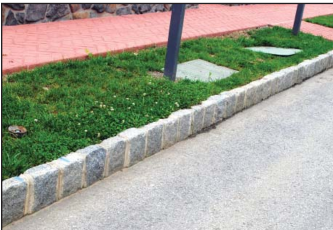
Belgium Block Curbing
