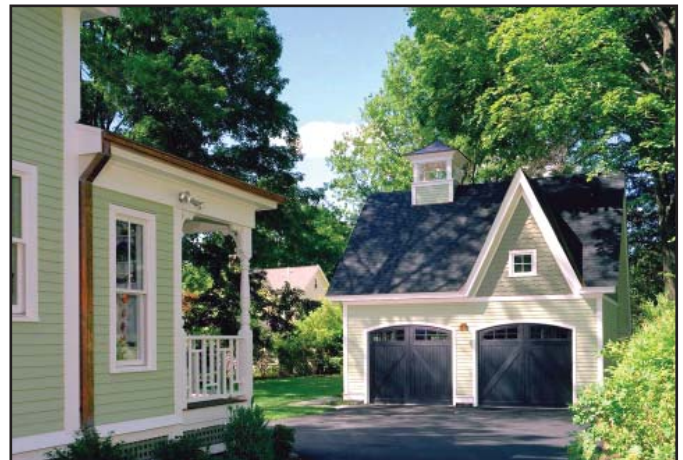
Garage setback from front facade of the dwelling
