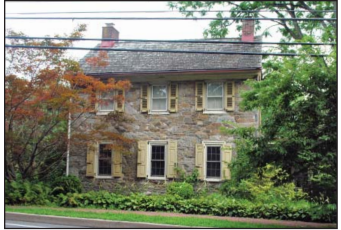
Traditional Building with traditional fenestration and materials
