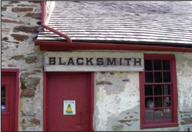
Old Blacksmith Shop
