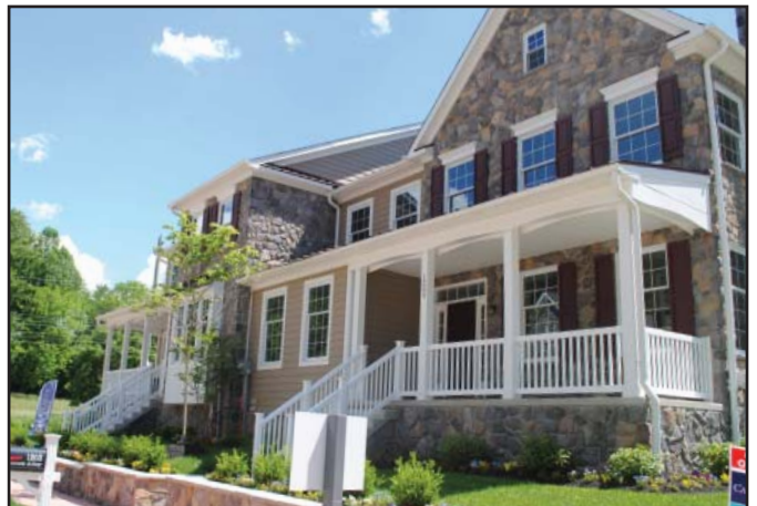
Infill Building with traditional fenestration
