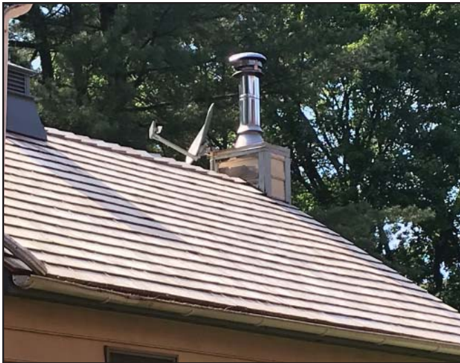
Satellite Dish Antenna located on the rear of the dwelling
