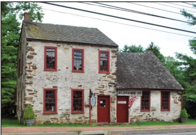
Traditional Building with varied roof lines
