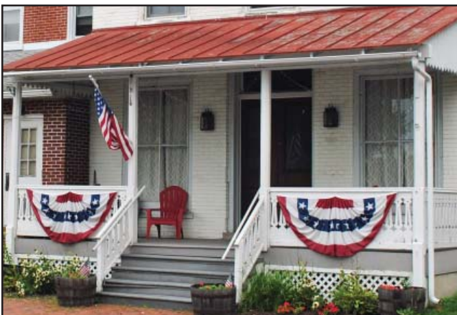
Front Porch with Lattice Skirt
