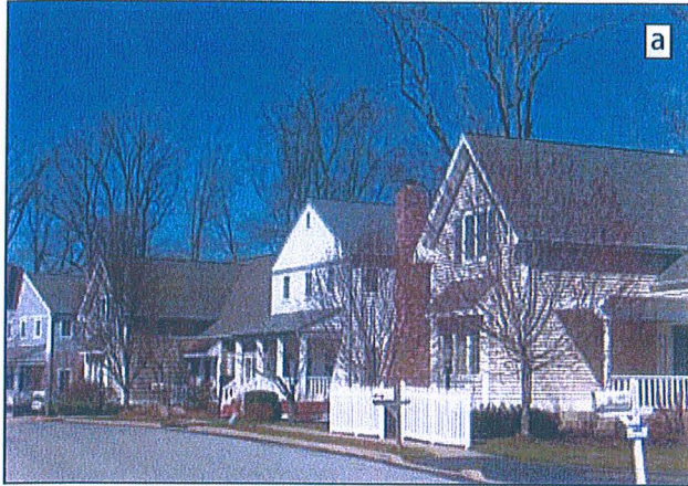
Eagleview TND - Dwellings along the Build-To Line
