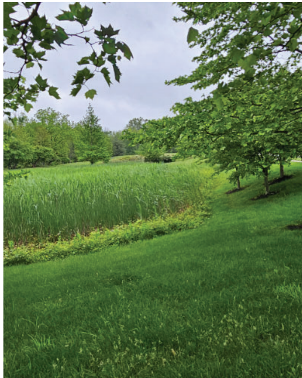
Bioretention, rain gardens, and other forms of vegetative stormwater management improvements are encouraged.
