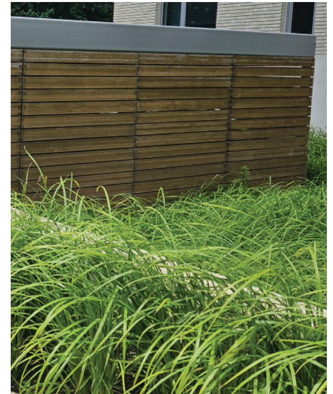
Decorative screen walls provide eight feet (8') or higher screening around three sides of the Ancillary Equipment.
