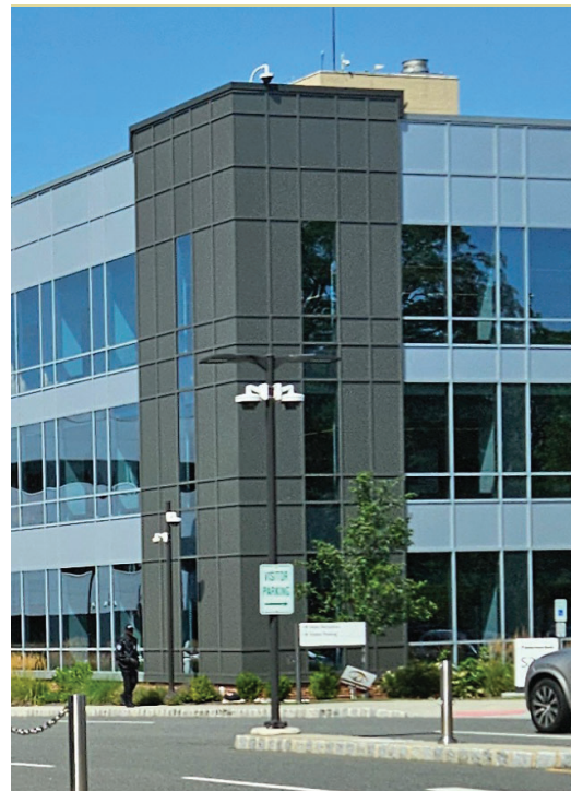
Each building with a Primary Facade shall have a defined building entry.
