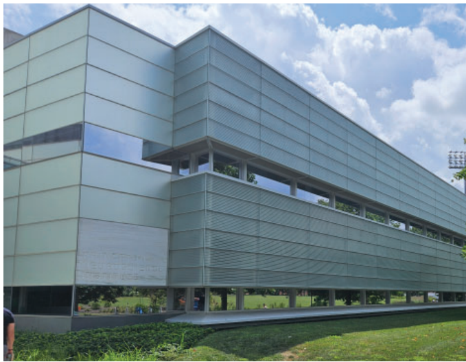
Primary Façades must have vertical breaks and avoid long, monotonous, uninterrupted walls or roof planes.
