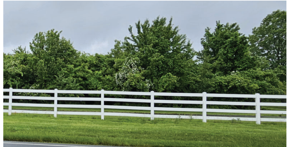
Split rail/horse rail decorative fencing shall be constructed parallel to the trail/walkway as a visual barrier and to provide consistency to the streetscape.
