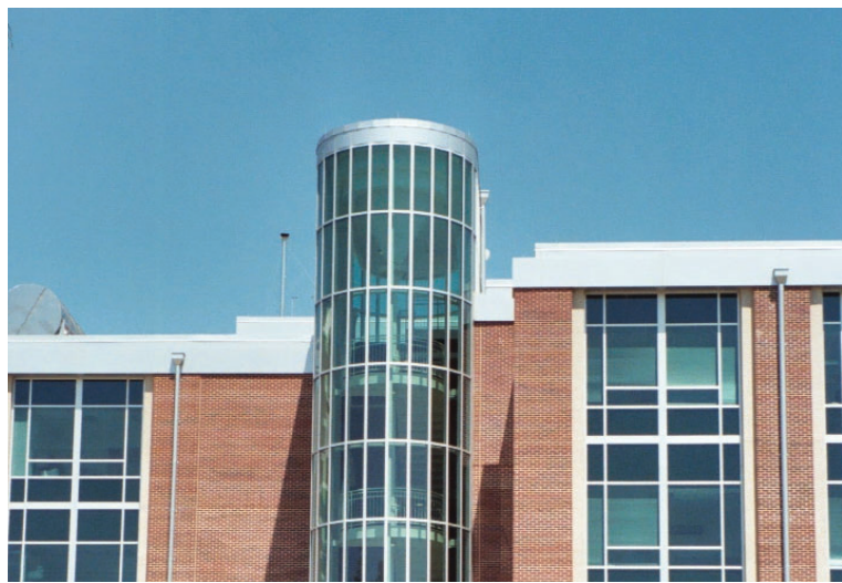
Primary Façades should have a defined base and cap with a change in material, color, and/or a projection to distinguish it from the main body of the façade.
