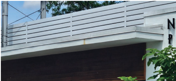
Caps on a Primary Façade shall include a decorative roof parapet to help visually screen rooftop equipment.
