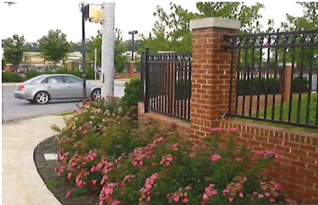
Pier-Fence-Hedge Combination enhancing the streetscape off-street parking
