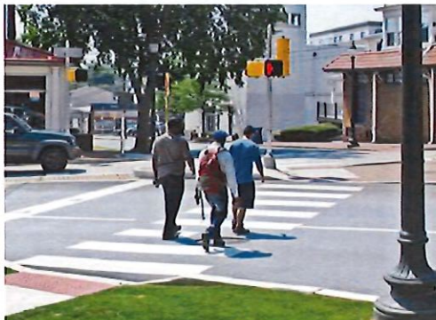
Crosswalks providing safe pedestrian circulation
