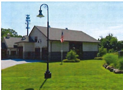
Existing Pedestrian scale Street Light at Fire Station
