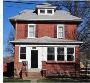
A successful example of an enclosed porch maintained the open areas (with windows) of the original porch
