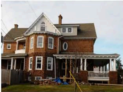
Brick and native building walls
