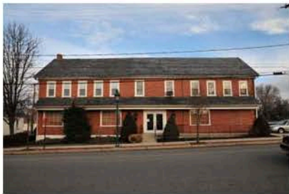
A more modern horizontal form that is successful because of good materials, acceptable window placement and proportion and the shed roof between the first and second floors.
