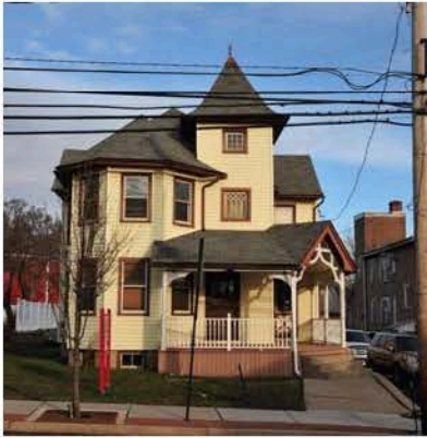
Vertical form is dominant in many of the older residential structures in the CBD
