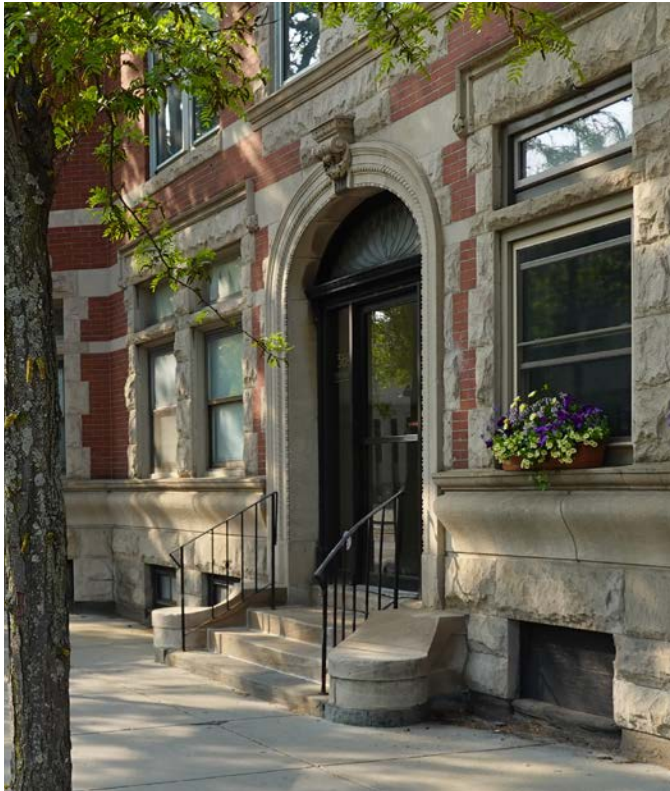
Example of recessed entry door to upper floor residential units.
