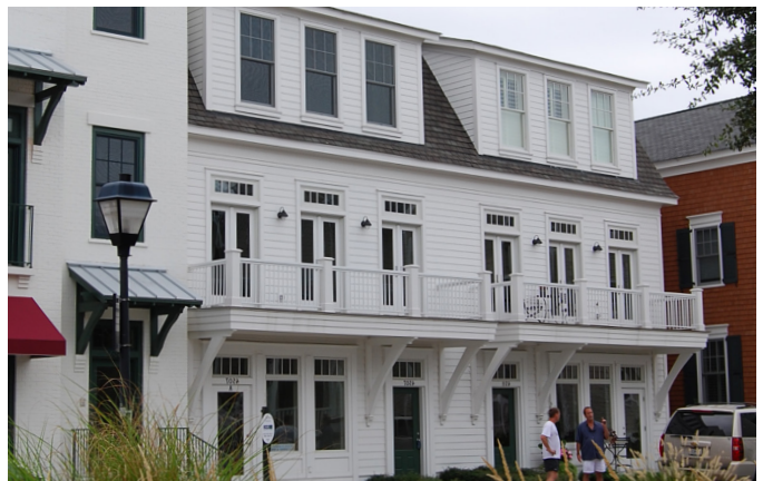
Example of house-scale building with sloped roof forms, shed dormers, wood and metal balconies, and wood siding exterior.
