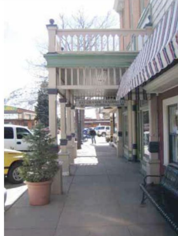
One-story gallery with shopfronts and uncovered balcony
