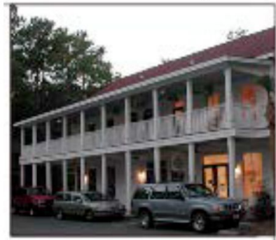
Two-story gallery with covered balcony
