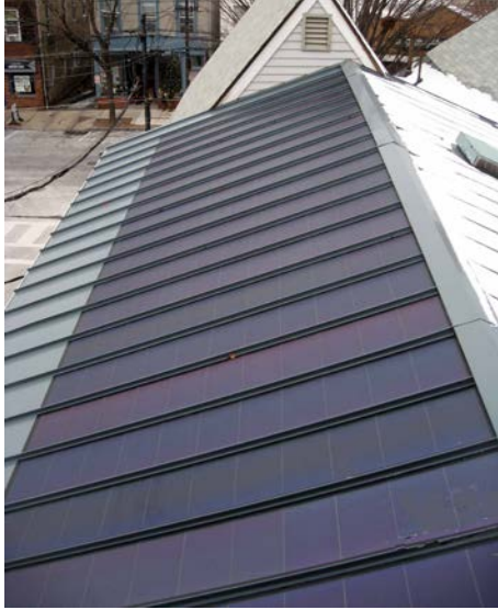
Laminated solar panels integral to roof (above) reduce visual impact by comparison to panels (below).
