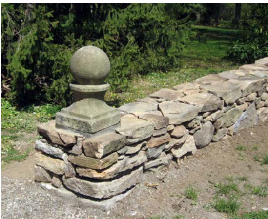
Front yard or entry drive treatment: dry-laid stone with an ornamental cast-stone or carved stone cap.
