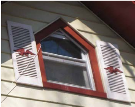
Above: correct installation of shutter and storm window; below: incorrect shutters.
