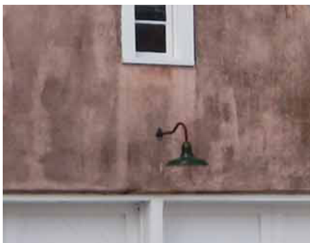
Graceful early to mid-20th c. style downlights can be lamped with LEDs and CFLs to be relatively efficient, and shielded for minimal glare and “Dark Sky” compliance .
