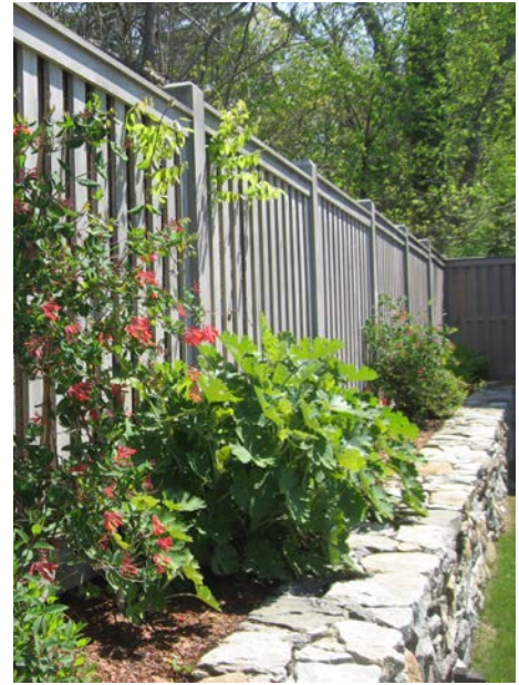
Low dry-laid wall provides excellent drainage for garden bed.
