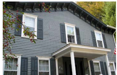
Narrow exposures (4") of clapboards add a rich texture and character to a facade.
