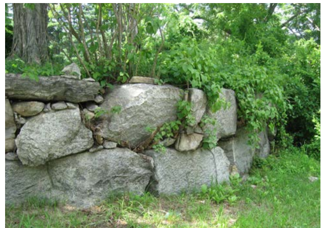
Traditional dry-laid gravity wall in a rustic style.
