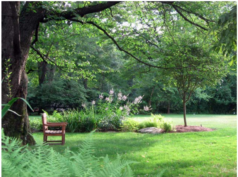
Rain Garden: 2/3 of roof runoff at this property is piped to a gravel reservoir beneath this garden
