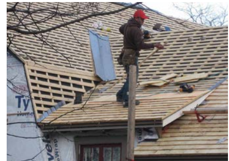
Traditional roof furring provides ventilation for shingles above.
