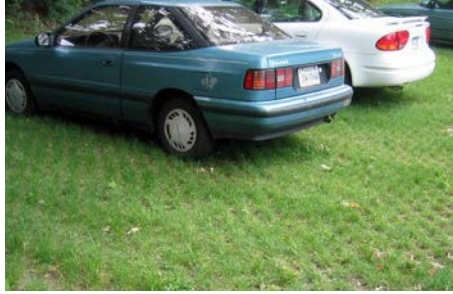
Open grid paving supports grass & stays green if use is light.
