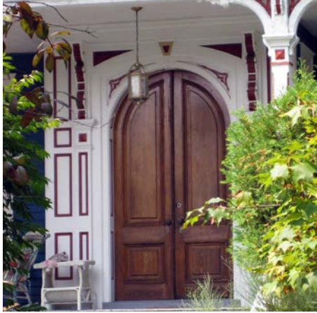
Successful entries consist of an assembly of elements including railing, step, molded surround and finally the doors themselves.
