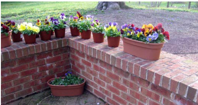
Mortared brick wall at sitting height with a brick coping.
