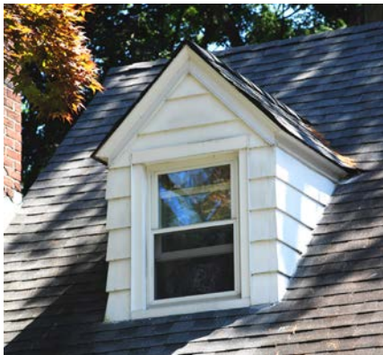
This traditional gable dormer has a good scale; the valley and sidewall flashings should be improved.
