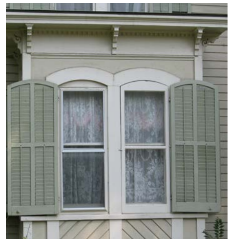
Shutters should follow the proportions in the diagram above, as in the example below.
