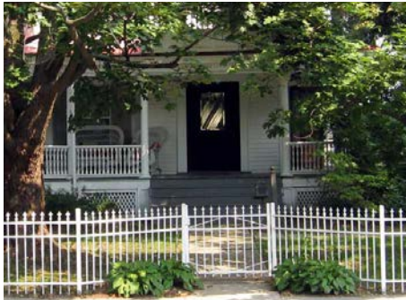
Metal fencing (above and below) is an attractive and durable pattern for more developed portions of the Village. It can be made of cast iron, wrought iron, steel or aluminum.
