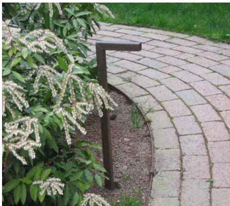
Low level, shielded lighting is best for path and landscape illumination.
