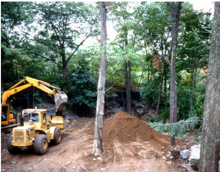
Misplaced fill (suffocating tree root systems) and construction activity killed all trees near this work.
