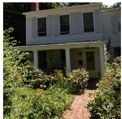
Porch shades the house, saving energy for cooling. Porous paving reduces runoff & recharges the aquifer.
