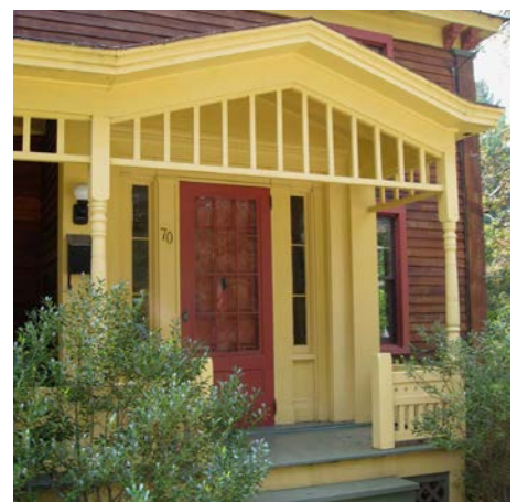
Red Hook has many great examples (above) of entrances that set patterns to be followed in new buildings.
