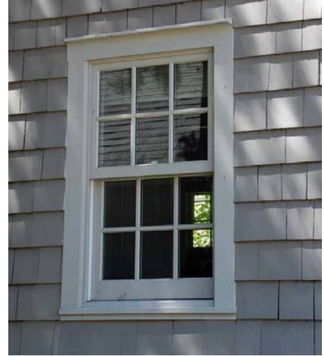
Above: a well-proportioned traditional double hung window, with head flashing, casing and sill.
