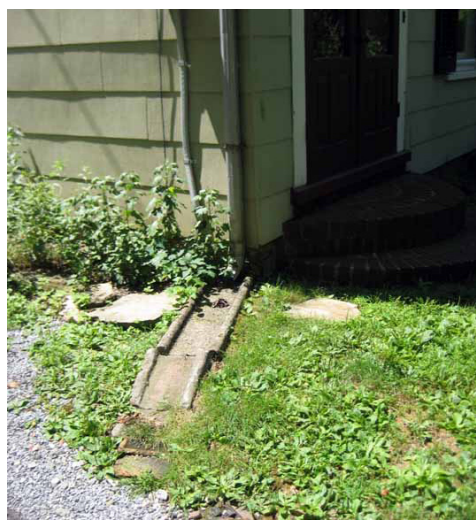
Unscreened splash block.
