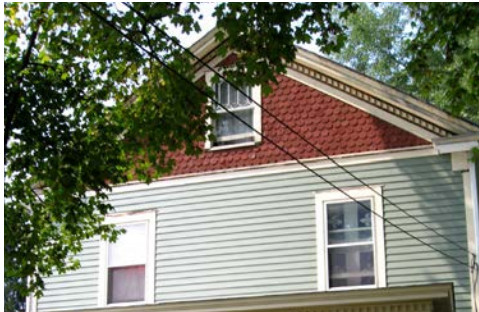
Clapboards are the prevailing siding material, occasionally complemented by fancy shingling, as in this "fish-scale" gable treatment.
