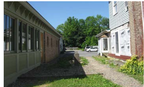
Passages to parking lots should be treated as improved public space, not neglected leftovers.
