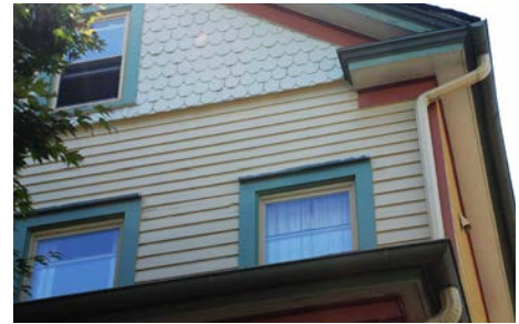
Well installed shingling and a carefully executed color scheme work together-note gutters and leaders painted to match siding & trim.
