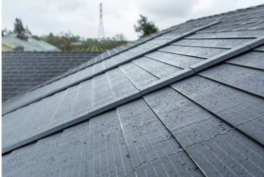
A roof with solar shingles; photo courtesy of GAF Energy
