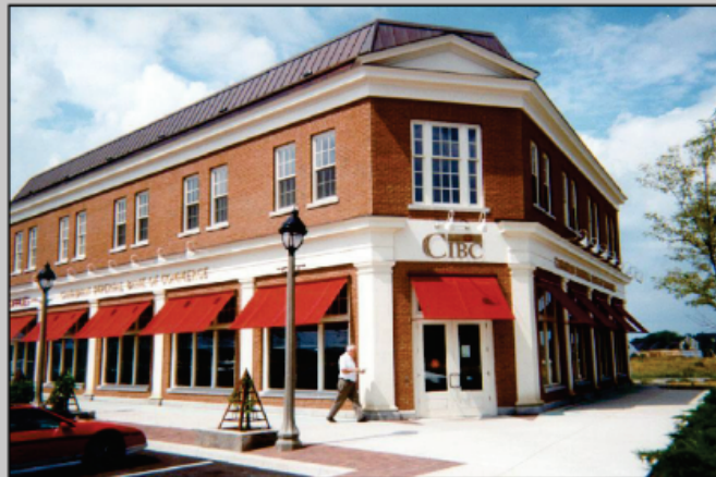
Example of High-Quality Façade Materials and Architectural Detailing
