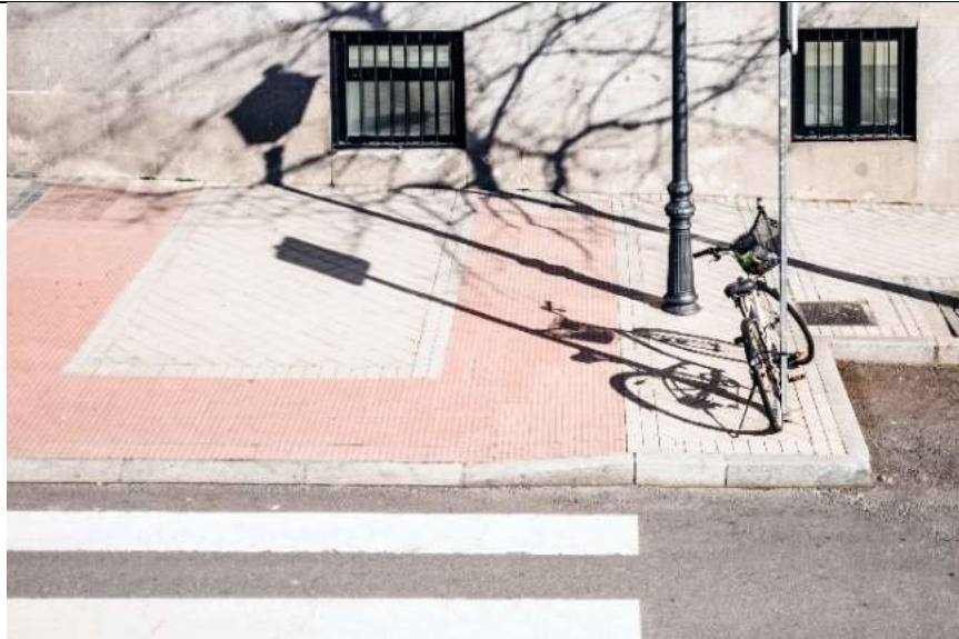
Pedestrian street crossing with a change in pavement to clearly delineate the crossing.
