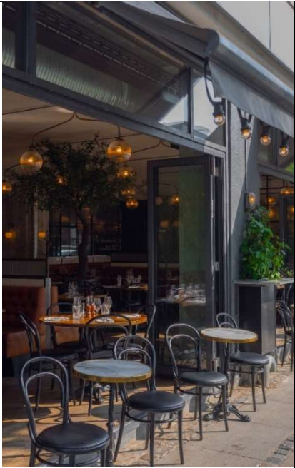
Retractable awning used for sidewalk seating area
