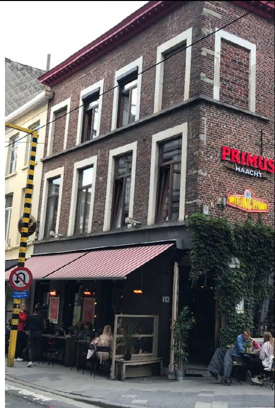
Example of mixed-use development with large windows, awnings, outdoor dining and signage suitable for HD-I and HD-II Subdistricts.
