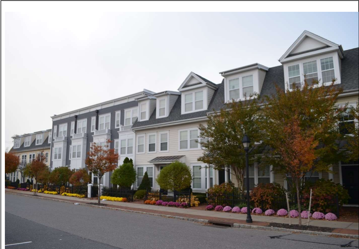
Example of varying rooflines with interesting architectural elements.
