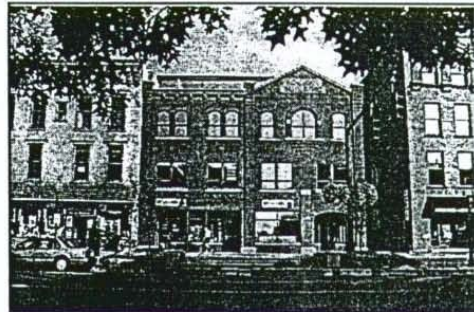
A new addition to the City of Saratoga Springs, the Roohan Building contributes well to the City's identity and is a good example of appropriate new construction.
