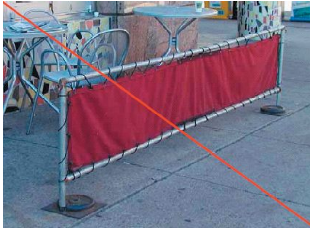
Figure 16. Prohibited pedestrian barrier.
