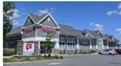
Figure 18. This is an example of a franchise business with building design elements and signage that incorporates many of the design standards desired for the TC District. Note rooflines, lighting, signage, bollards, side parking, side entrance and windows.
