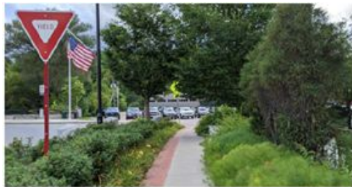
Figure 4. Example of a landscaped sidewalk used in part for screening a parking area.
