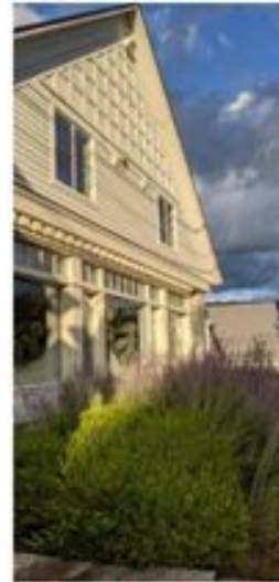
Figure 16. This is an example of facade windows that meet the design standards for the TC District.
