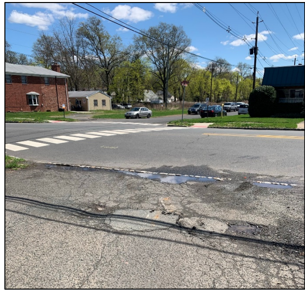
Picture 8 – Ingress/Egress on East Second Street.
