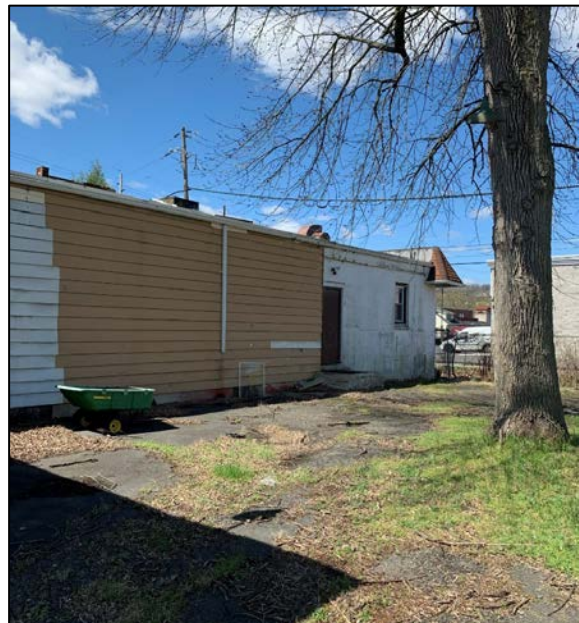
Picture 4 – Rear elevation of existing commercial building.
