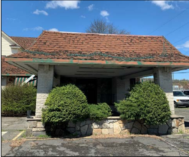
Picture 1 – Front of existing commercial structure facing inner parking lot.
