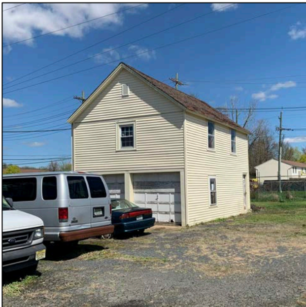
Picture 3 – Accessory Structure behind existing building along rear lot line.
