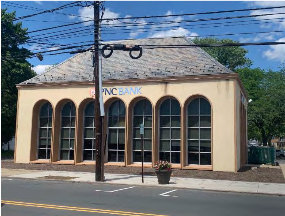
Figure 4 – Adjacent Lot 9.01, PNC Bank, from Park Avenue
