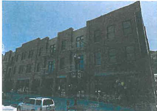
The Sawyer Building at 125 W. Broadway
