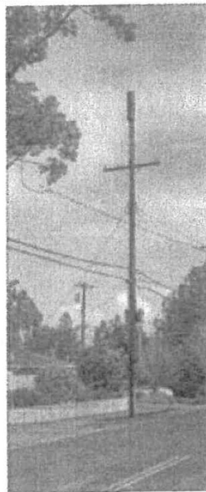
Figure 5: Installation on a Utility Pole
