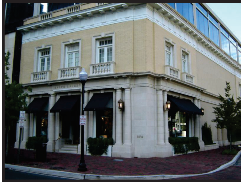
Figure 17: Example of a building utilizing several façade materials such as cast stone, glass and stucco and containing architectural details such as cornice and moldings, recessed doorway, awning and belt course
