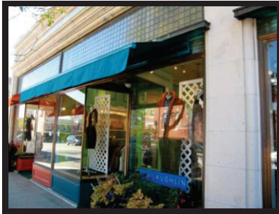
Retractable awning located below transom
