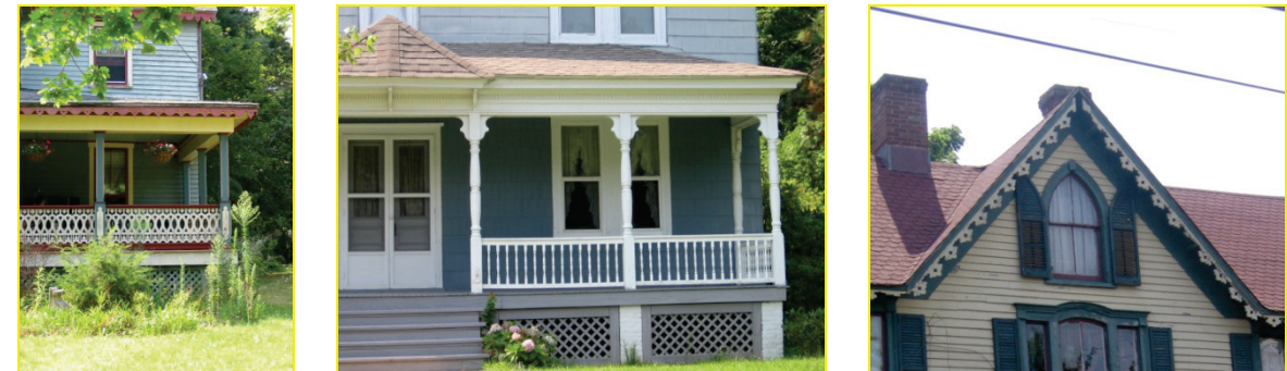
Figure 12: Examples of ornamentation, columns, railing, chimneys and trim details
