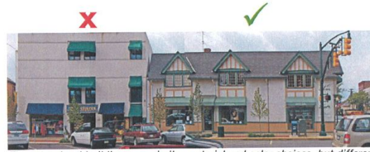
These two local buildings use similar material and color choices, but different massing and detailing strategies. The structure to the right demonstrates the preferred approach towards massing—using vertically-oriented bays, glazing, materials and colors to break up the horizontal facade
