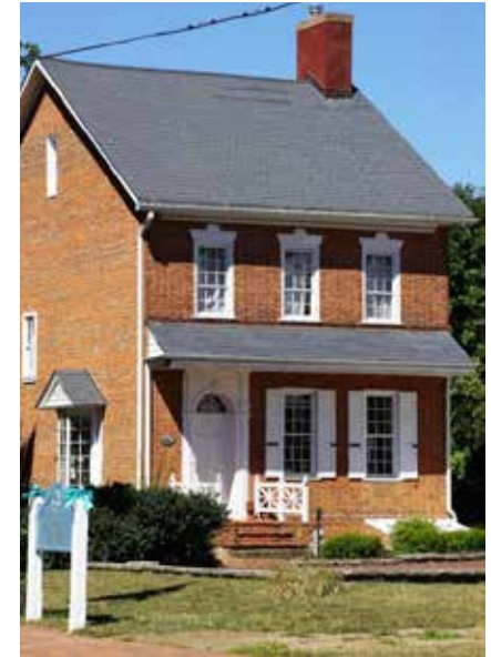
Hulse House Brick Exterior
