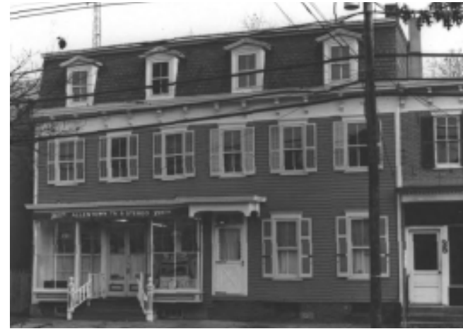
S. Robbins House and Store, 23 South Main Street
