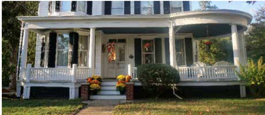
Well preserved wrap around front porch
