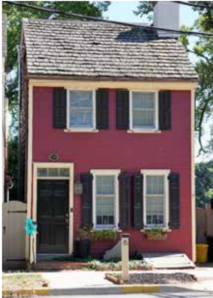
Peter Bruhere House Wood Clapboard Siding
