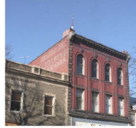
APPLICATION: Antenna Chimney | LOCATION: Frederick, Maryland DESCRIPTION: 2' tall, 1' x 1' x 1'
