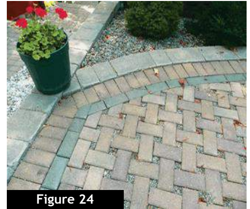
Figure 24 Porous pavements are encouraged to further facilitate infiltration and slow storm water runoff. These materials are especially useful along the periphery of parking areas and/or adjacent to bioretention areas (below).
