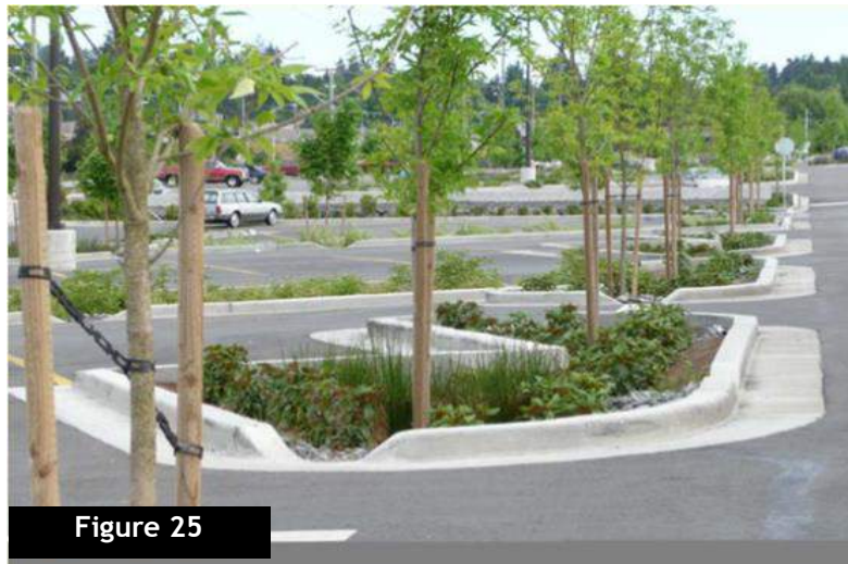
Figure 25 Where appropriate, bioretention areas and bioswales similar to the above may be used to promote the infiltration of storm water. These installations would be appropriate in parking lot medians or in linear strips along drive aisles or behind parking lots in lieu of large, unsightly retention facilities.
