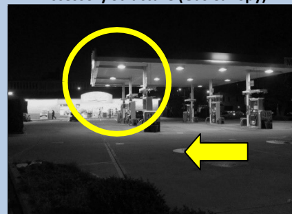
Accessory Structure (Gas Canopy)
