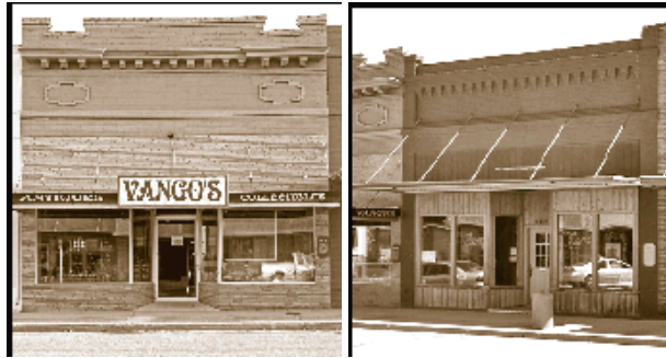
Figure 7. The Weiland Building (left) and the August Krause Building are prime examples of maintaining original character with similar scale/building heights.
