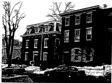
Roofline Dormers add architectural detail and interest to building facades.
