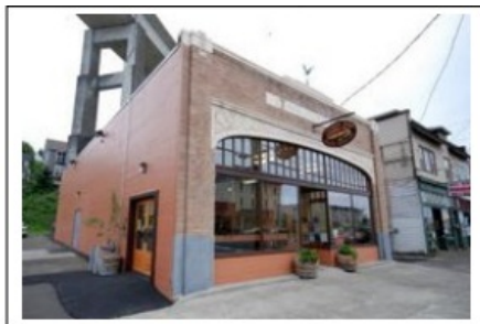
Figure 14.195-10: Non-Industrial Building, Flat Roof Behind Parapet Wall
