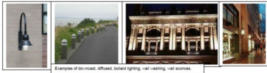
Figure 14.195-20: Downward and Diffused Lighting, Wall-Washing Lighting
