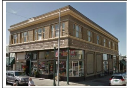
Figure 14.115-2.b: Base, Middle, Top of Building
