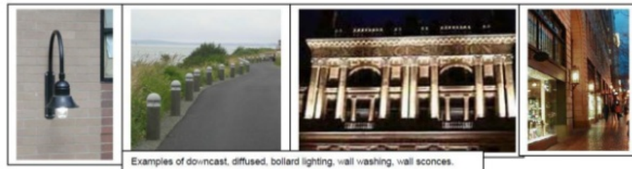
Figure 14.158-16: Downward and Diffused Lighting, Wall-Washing Lighting
