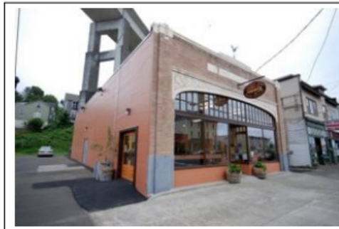
Figure 14.115-5: Non-Industrial Building, Flat Roof Behind Parapet Wall
