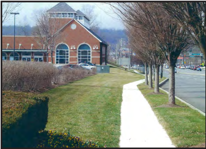
Streetscape with Street Wall formed by Retail Building located close to the sidewalk.
