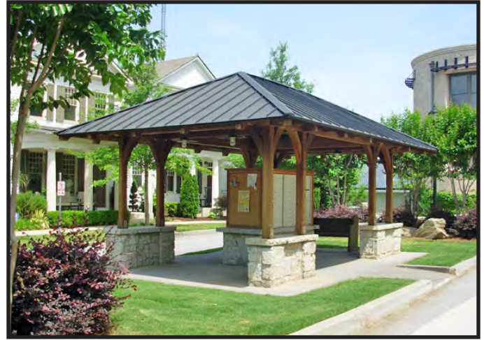
A covered common mail area with community message board, bench, and integrated sitting walls.
