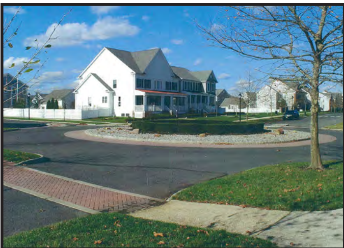
A decorative crosswalk contrasts with the cartway surface in order to promote visibility.
