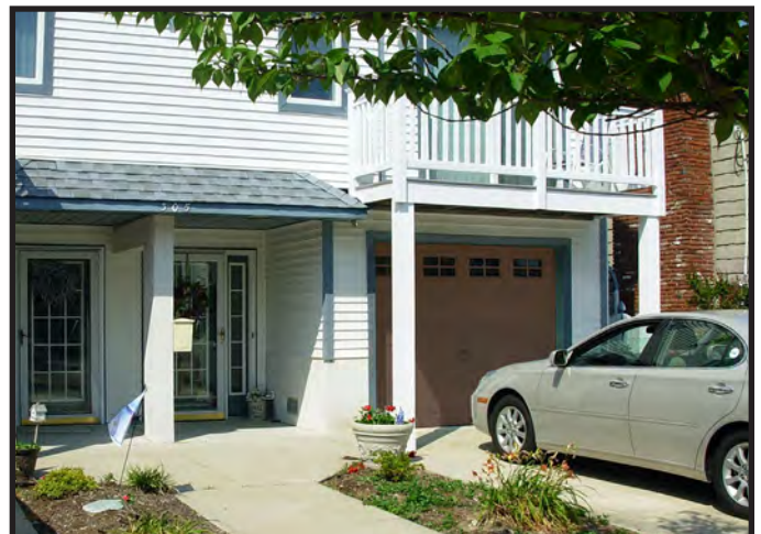
Recessed, non-white garage door helps to minimize the appearance of the front-loaded garage.
