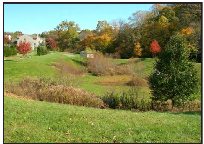
Naturalized Stormwater Basin with indigenous plants.
