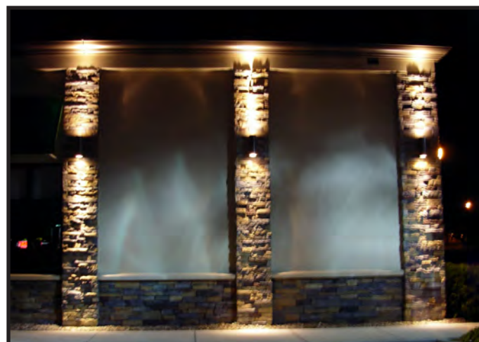
Wall lights complement the building architecture by accenting the piers.
