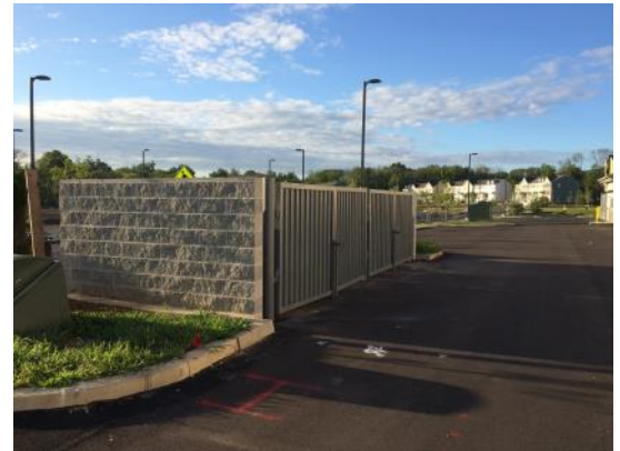
Example trash enclosure - Valley Gate , Warrington, PA
