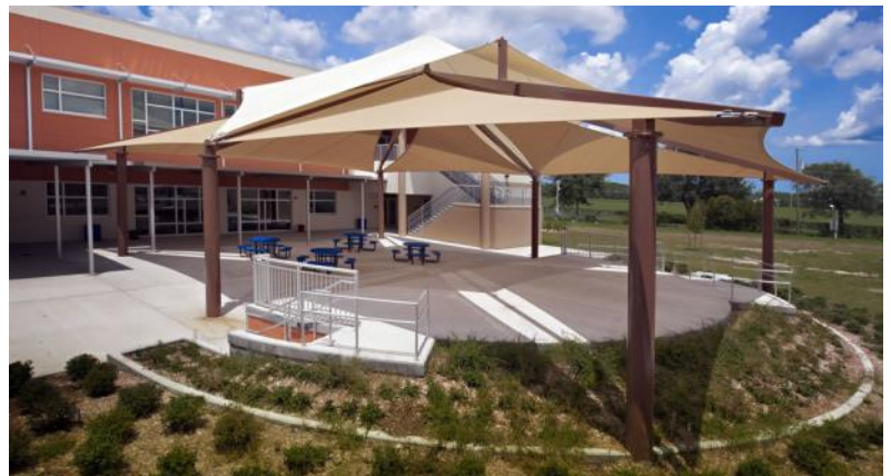
Example Shade Systems Inc. - Multi-level framed sail structure
