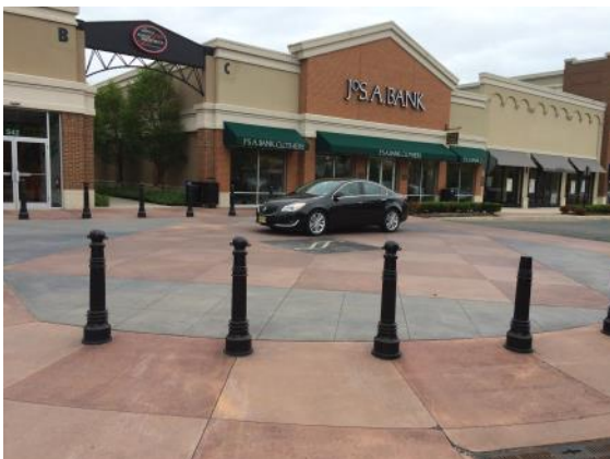
Metal bollards - the Shoppes at North Brunswick, North Brunswick , NJ
