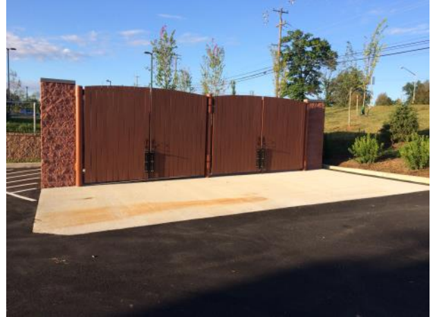
Example trash enclosure - Valley Gate , Warrington, PA
