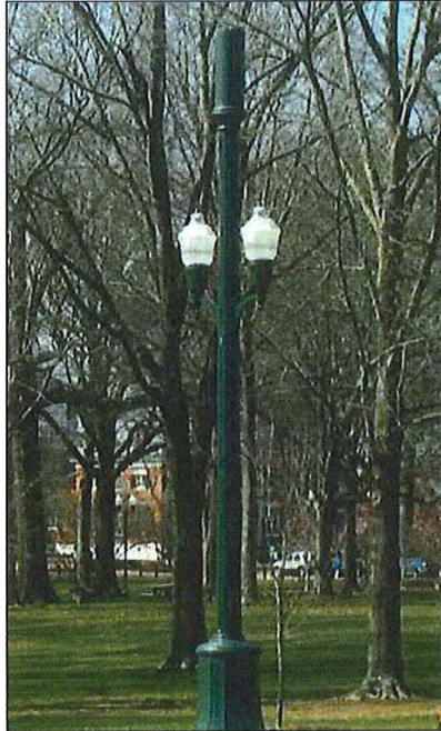
Extension of Existing Street Light
