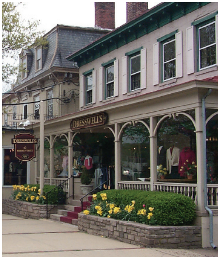
The commercial building above on Bridge Street is a Federal style building with a front porch addition designed in an Italianate style.
