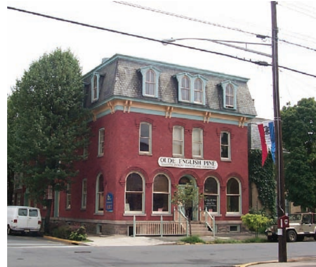
A commercial building on North Union Street.
