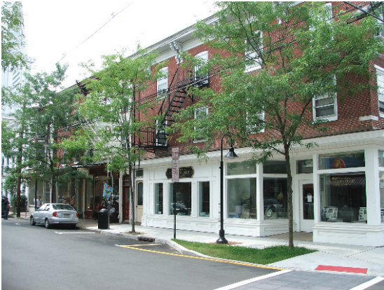
This North Union Street building was recently rehabilitated to accommodate new uses. The design of the storefront is consistent with the front windows and transoms of that period.
