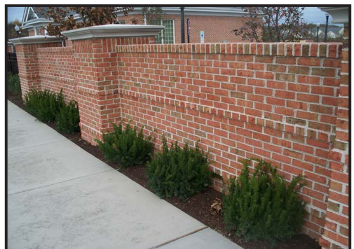
Solid Brick Street Wall at Street Intersection, ESB Bank Cranberry Township
