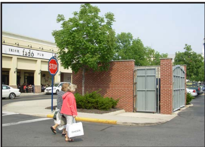
Attractively Enclosed Dumpster Area, Easton Town Center, Columbus, OH
