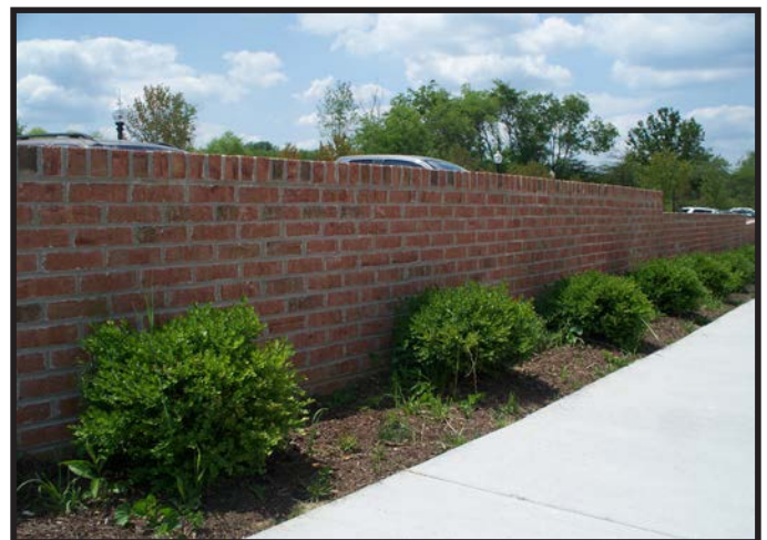
Solid Low Brick Street Wall, BelleVue Commons, Cranberry Township
