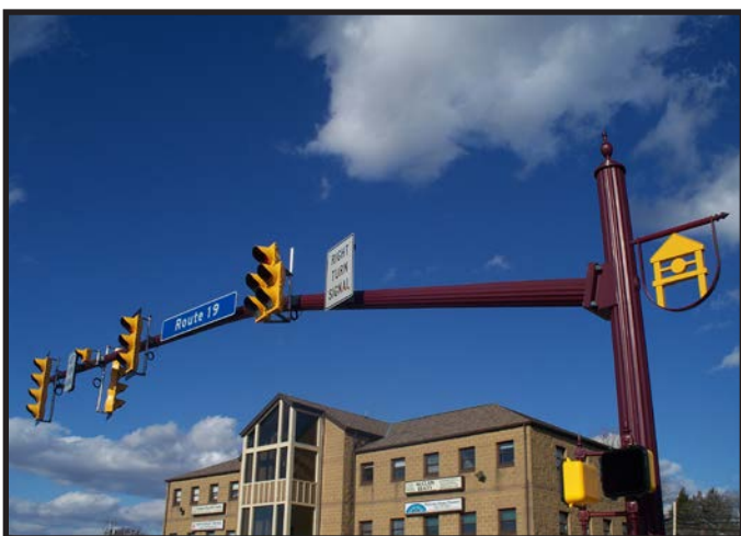
Decorative Traffic Signal, Hartners Drive at Route 19, Cranberry Township
