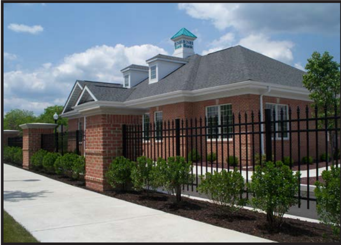
Brick Piers and Black Fence form the Street Wall at ESB Bank, Rochester Road, Cranberry Township
