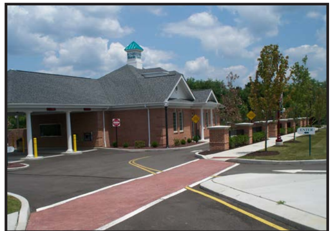
Crosswalk in Driveway Throat, ESB Bank, Cranberry Township
