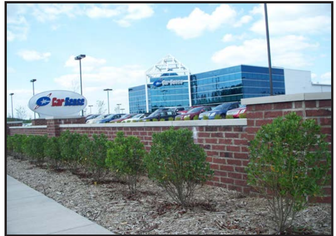
Street Wall, Car Sense, Route 19, Cranberry Township
