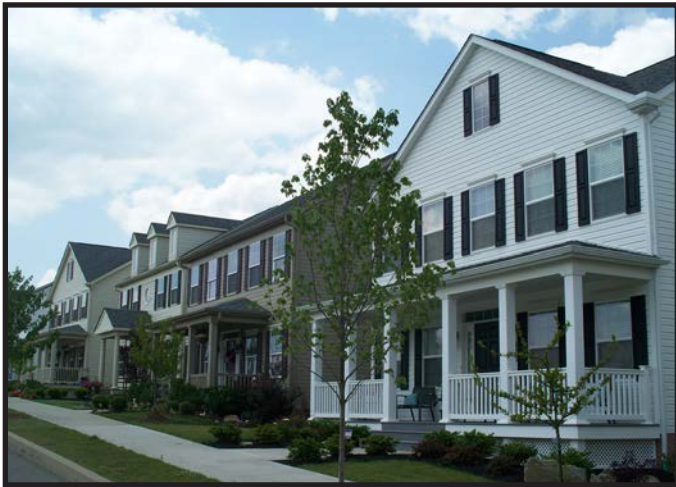
Concrete Sidewalk with Grass Strip, BelleVue Park, Cranberry Township
