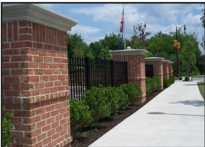
Street Wall with Brick Piers, Black Fence, and Shrubs, at mid-block parking lot location, ESB Bank, Cranberry Township
