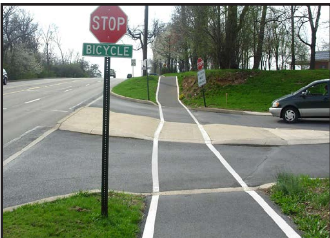
Grass Strip Separates Bike Path from Roadway
