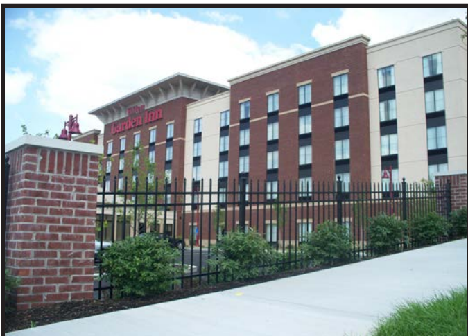
Street Wall, Village of Cranberry Woods, Cranberry Township
