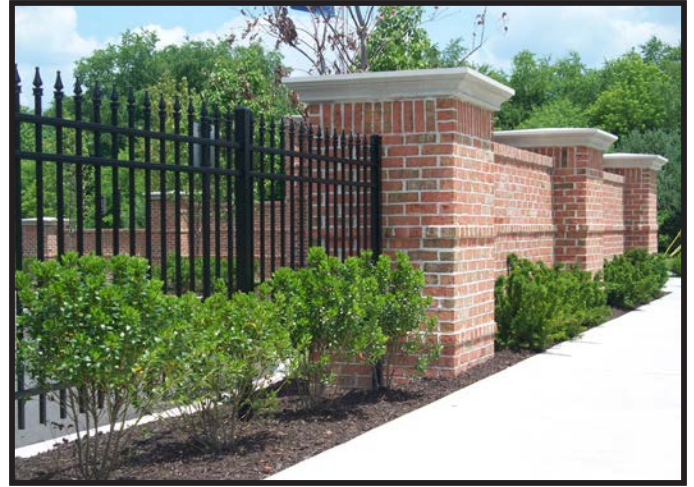
Street Wall: Rochester Road, Cranberry Township
